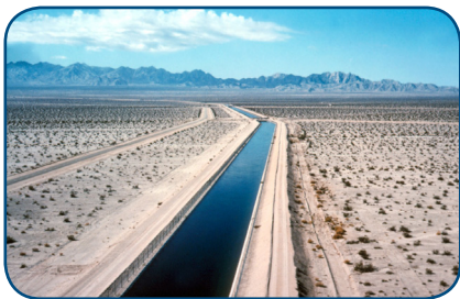
Colorado River Aqueduct
