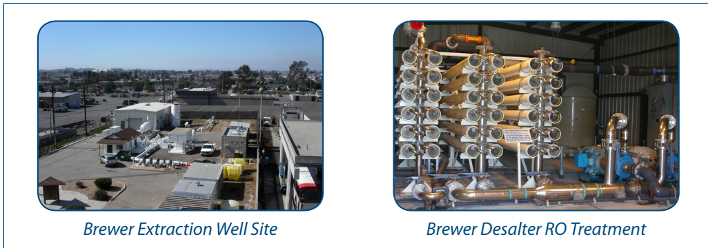
Figure 10-4: Brewer Desalter Facility Equipment
